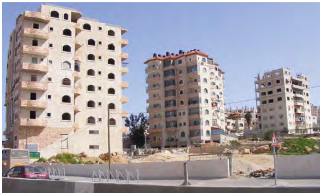
Picture 3.4: Kafr 'Aqab New Building Construction
